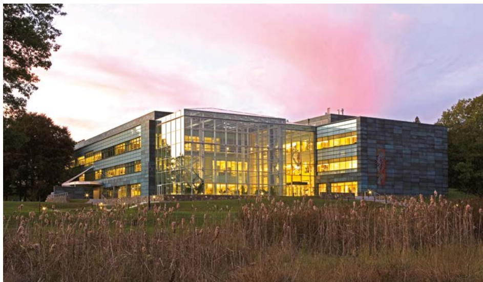
NEB Headquarters in Ipswich, MA, is LEED-certified and designed with sustainability in mind.
